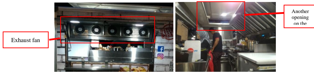
Figure 7: Air Ventilation in Food Truck Chef Pak Cik Kluang (FT-Q)
